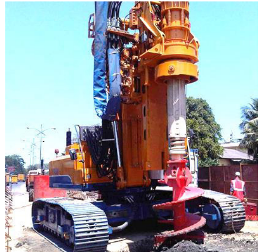
Figure 3.4 : Hydraulic Piling Rig
